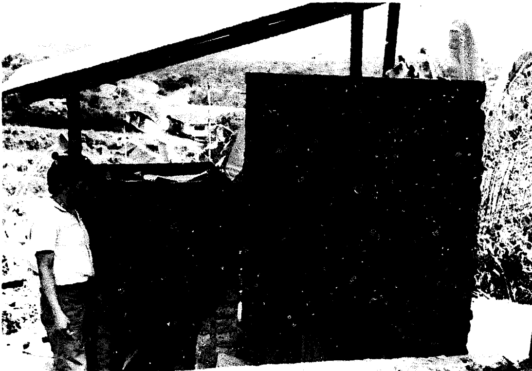
Photo 10. A suitable smoking room, with smoke channelled in from outside.
