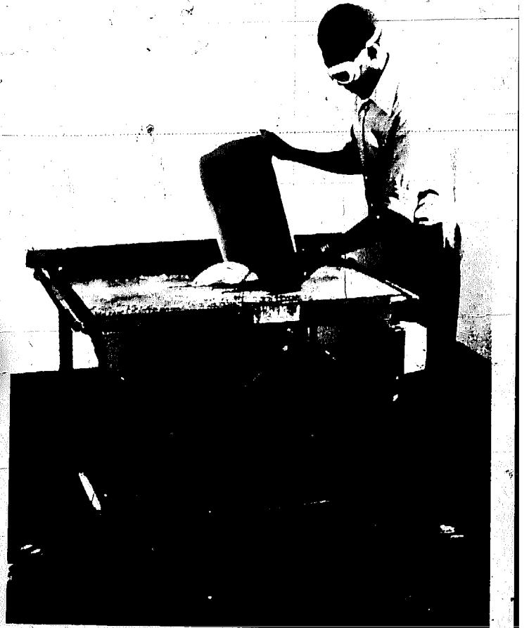
FIGURE 15: Cutting scrap on a circular saw.
