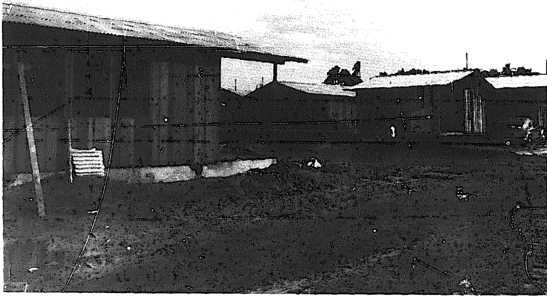
Photo 3. View of houses nearing completion. In the foreground, house with ceramic block foundation and cement floor
