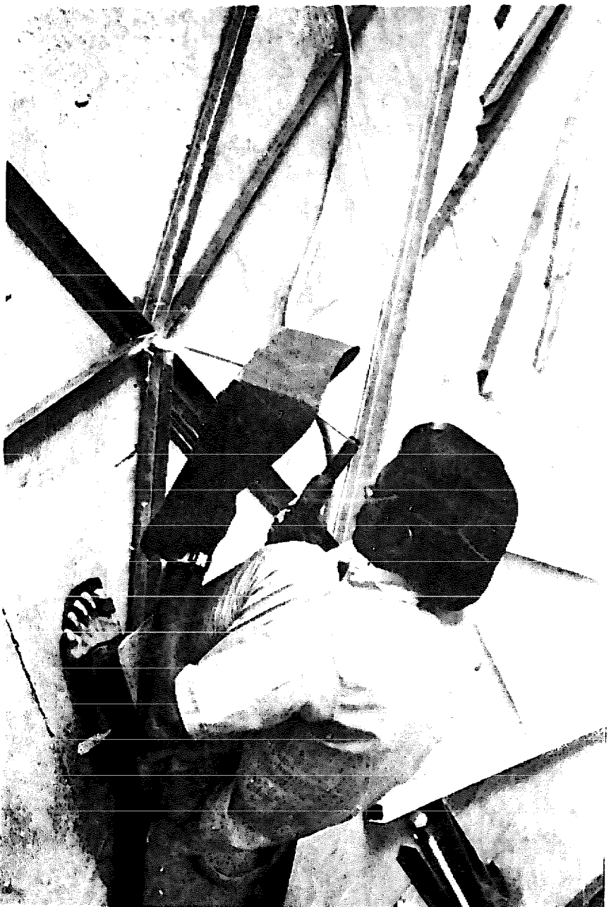
A 12 PM P.M. - tower half is composed and welded.
