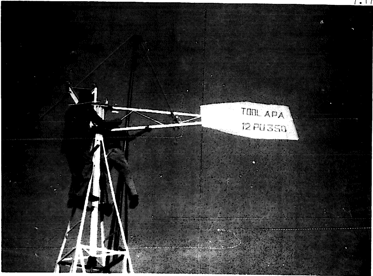
Installing a 12 PU 350 head construction
