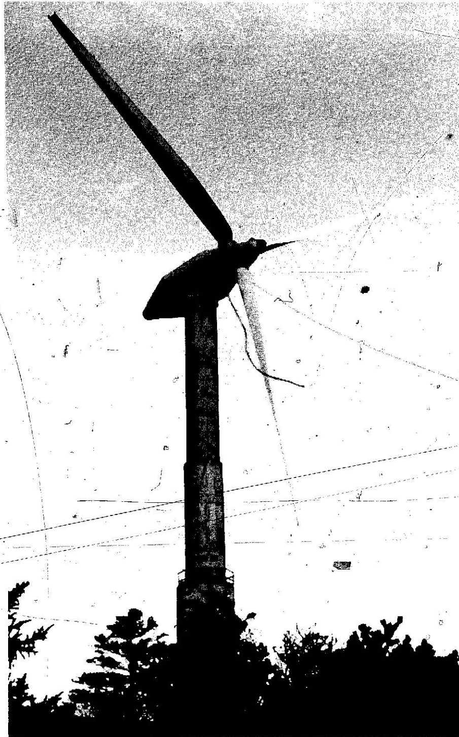
The 2000-kW wind machine at the Tvind School in Denmark. This machine supplies both heat and electricity to the school.
