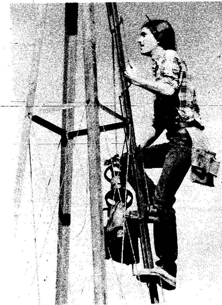
The reconditioned water-pumper at the Park ranch was carried aloft piece by piece and reassembled at the top of the tower.
