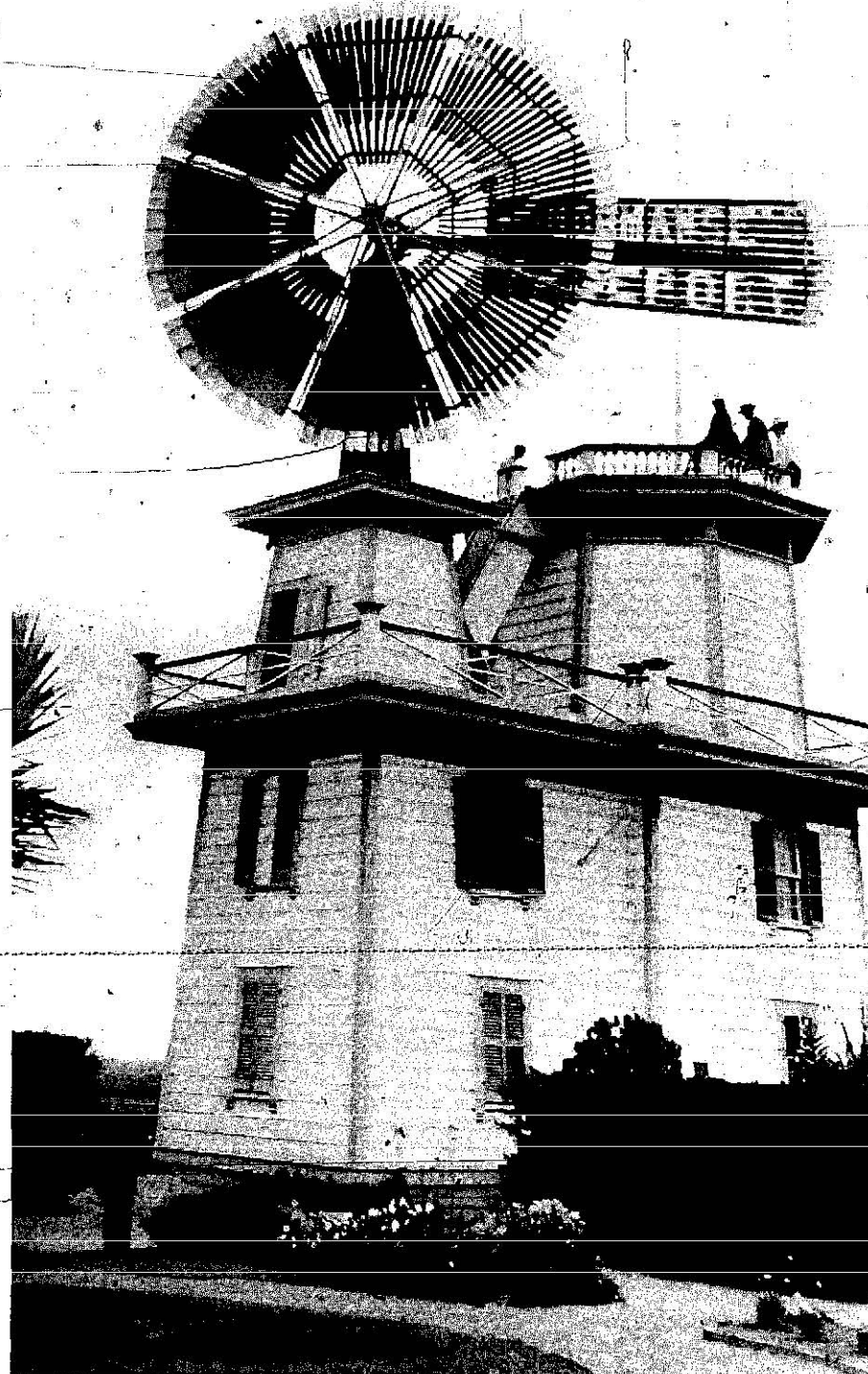
A water-pumping windmill of early California. The storage tank was built into the structure itself.
