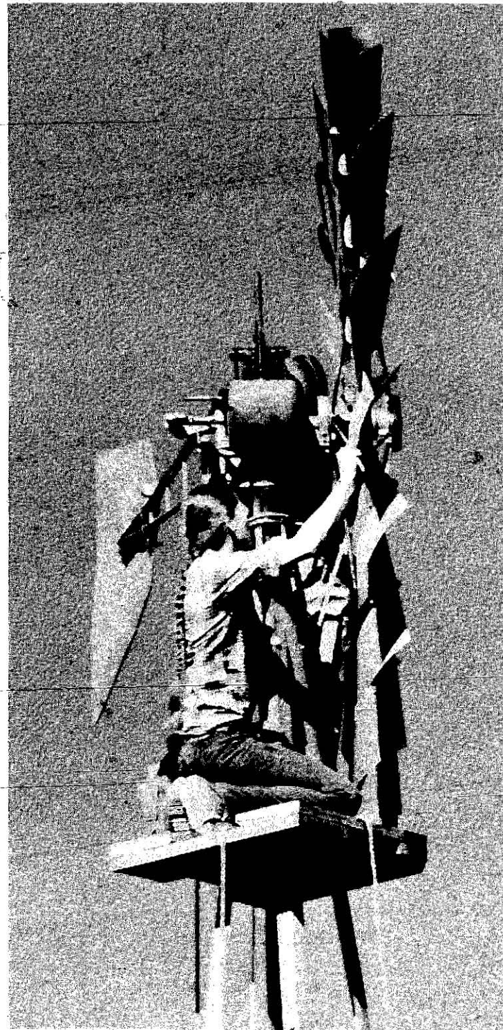
American Farm windmill in final stages of assembly.
