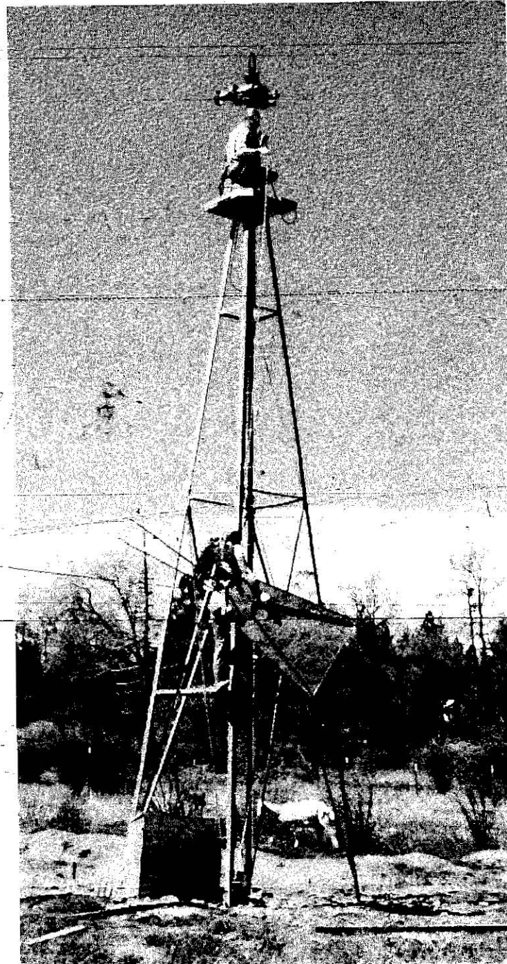
The reconditioned water-pumper at the Park ranch was carried aloft piece by piece and reassembled at the top of the tower.
