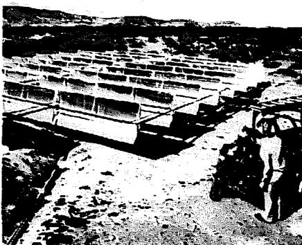
**SOLAR THERMAL ELECTRIC** research is being carried out on both large and small installations. Shown here is a 4 KW capacity array of concentrator collectors which heat a fluid that drives a turbine generator. The variable output of the array is fed into the AC service of the laboratory through a Gemini Synchronous Inverter. The future looks promising for solar thermal electric installations where insolation levels are high as is typical of the Southwest part of this country.
