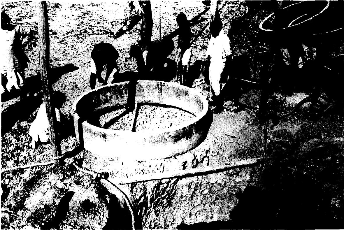
Fig. 5. Pre-cast concrete rings for lining a well in Bihar, India. (photo: Jim Cranmer/Oxfam.)
