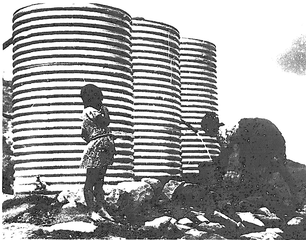
Fig. 19. Storage tanks for a village water supply in Lesotho (photo: Associated Newspapers Group Ltd.)
