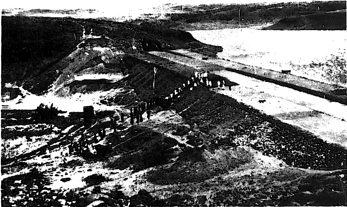
Fig. 10. Percolation dam being built in the Maharashtra state of India, December 1969. Construction was by manual labour paid for on a food-for-work basis.
