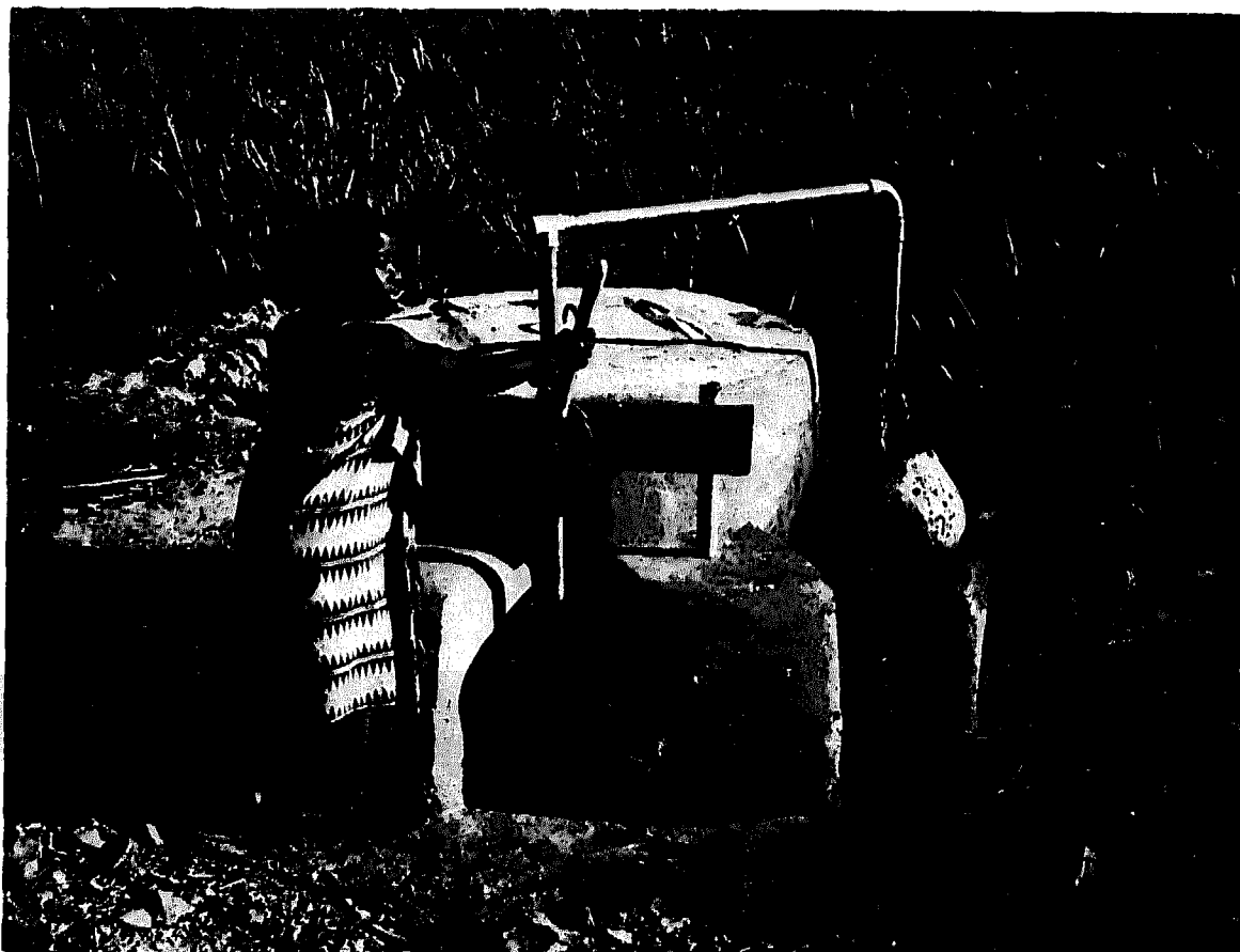
Fig. 6. A shallow well in Tanzania with the top closed to prevent pollution and with access to water only by means of a pump. But semi-rotary pumps at village wells have a poor record for reliability, and this one has been set up with little regard to ergonomics, as can be seen from the stance of the operator. So two out of three criteria for technical appropriateness are not satisfied. (photo: Oxfam).
