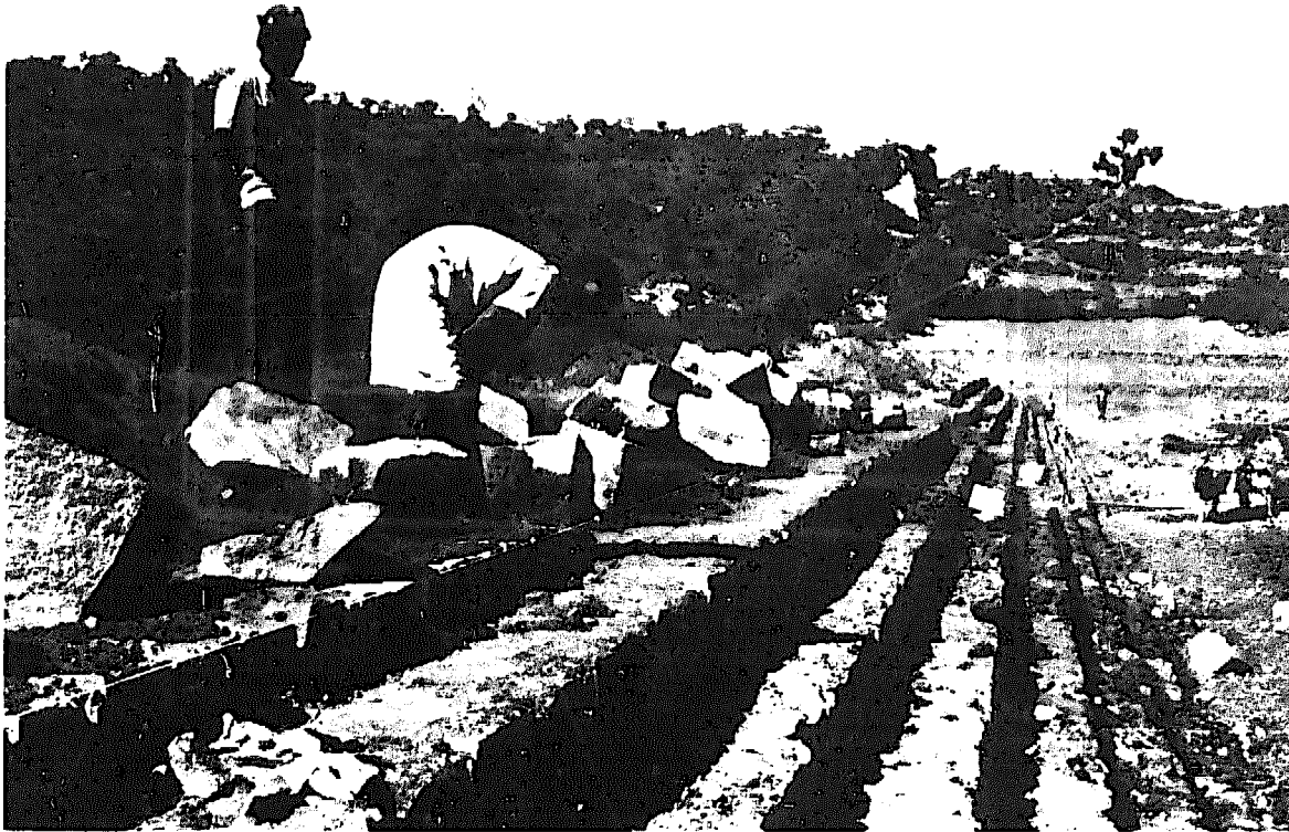
Fig. 11. Stone-faced earth dam for water conservation under construction at Otterthotti, in the Karnataka state of India. (photo: Father Godest).
