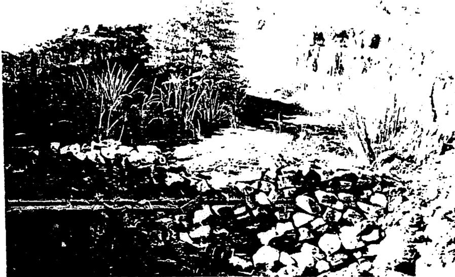
digging into the soil and causing damage. It also helps to check the fast-flowing water from washing away soil. This structure must, however, be loose so that water may easily pass through the stones.
