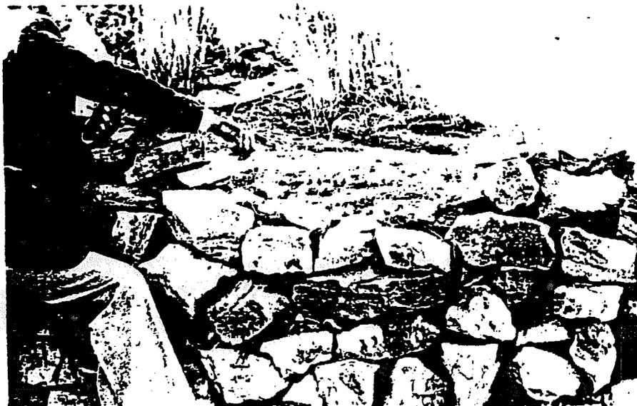
allow running water to pass through. Unless you allow for this outlet, the force of the water will break and wash away your structure.
