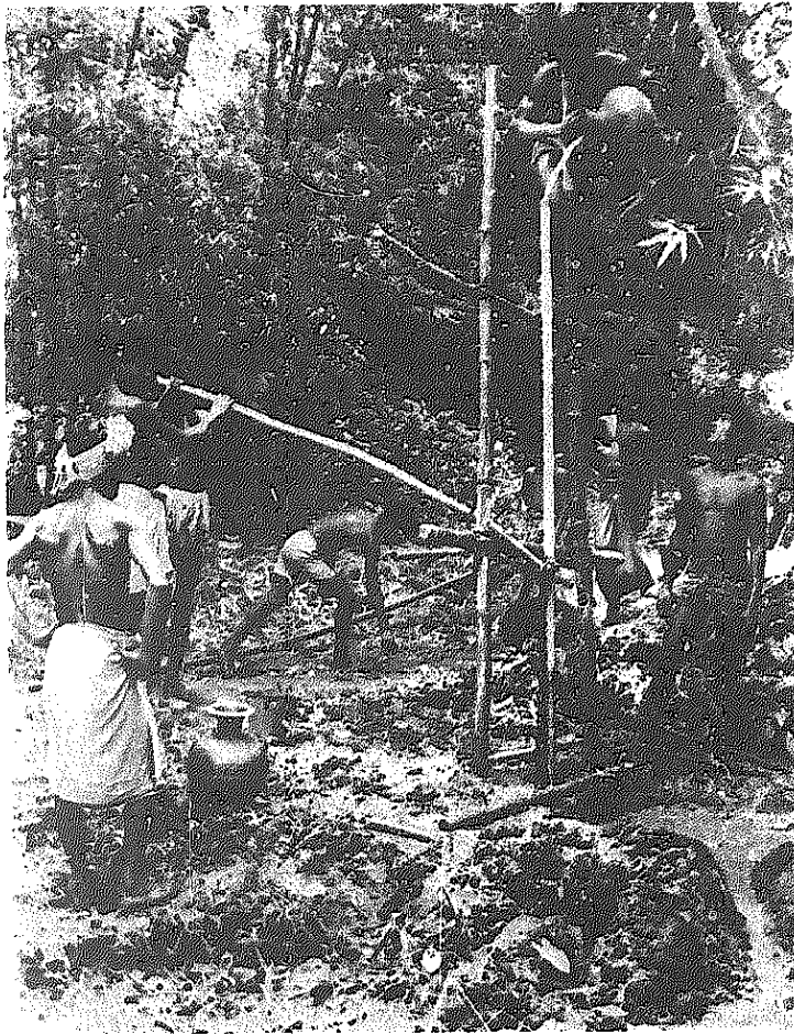
Sinking a tubewell
