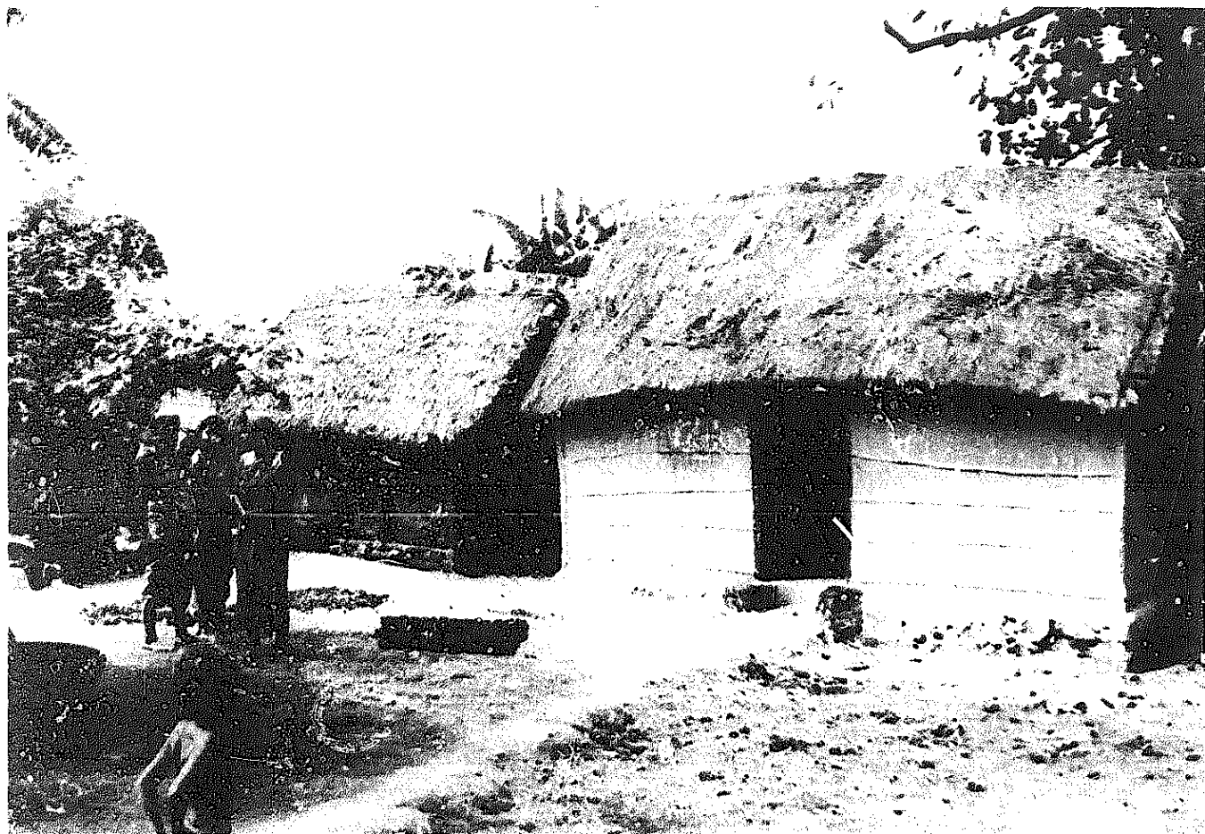
A typical village home with walls made of jute sticks and a thatched roof of rice straw
